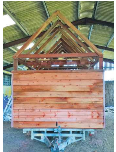
Pegs, as seen in the roof trusses, hold the frame together
